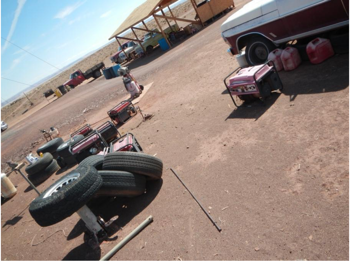
Image 2: This photo shows seven generators beside one of the host homes. As generators fail, families need to replace them quickly in order to continue receiving critical energy services for their homes. Frequent generator failure, added to fuel costs, results in an expensive and inefficient home energy system. Photo: AGCI.
