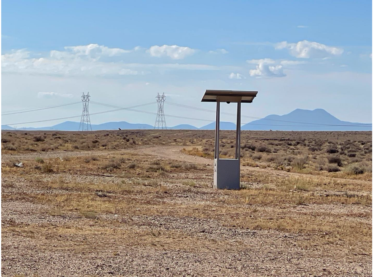
Image 4: Installed Solar Station (foreground) with power lines in the back. Although the power lines are located close to the rural host families in this project, transmission lines are not built to connect these households to the grid. Photo: SkyHook Solar.
